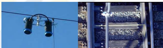
Camera switch inspection by Damill(S) continuous view of status important or remote switches (Deliverable 3.2 p 23)
